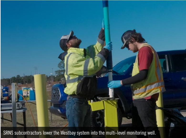
SRNS subcontractors lower the Westbay system into the multi-level monitoring well.
